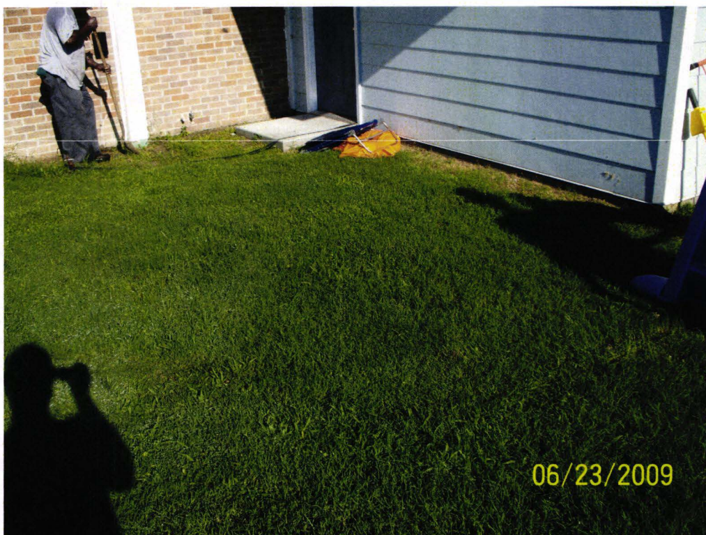
Picture 1: Location of UST 1137Iris prior to excavation.
