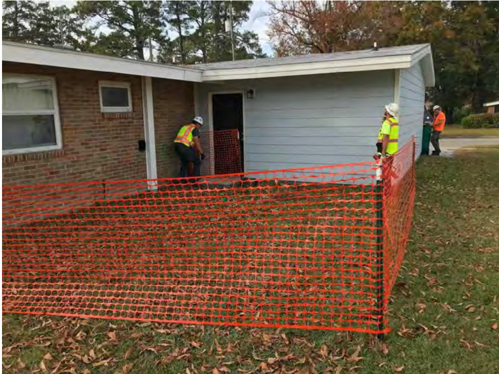
Photo 1: Tank Site Location
