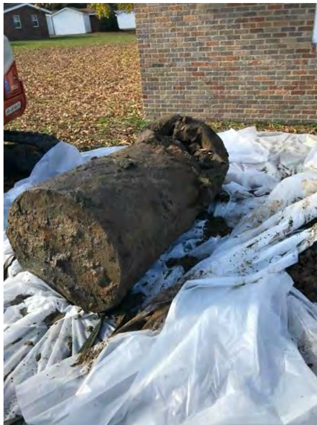
Photo 2: Tank Removed
